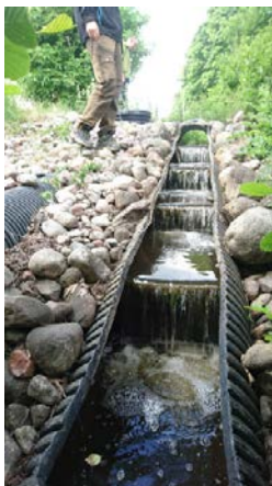
a. The old fish pass. Migration obstacle at low flow conditions.
