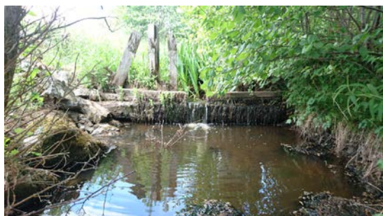
c. Wooden weir upstream the fish pass. Migration obstacle at low flow conditions
