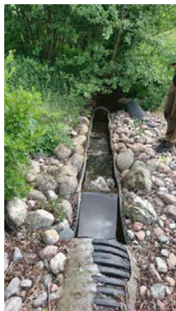
a. The old fish pass. Migration obstacle at low flow conditions.
